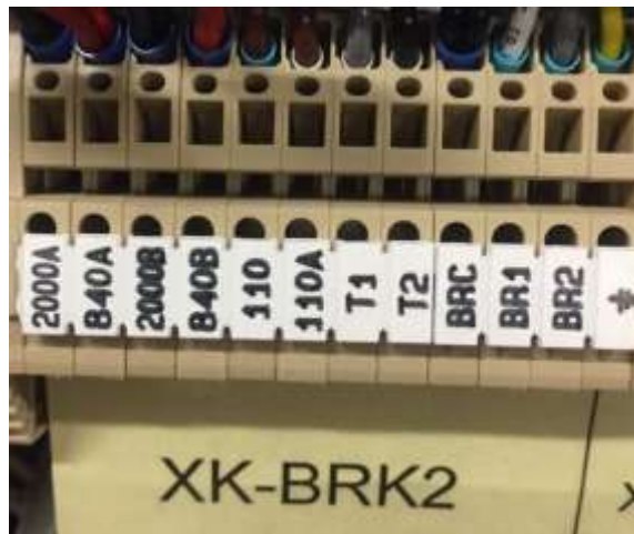
Figure 6-Brake and Micro Switches Connection Terminals
